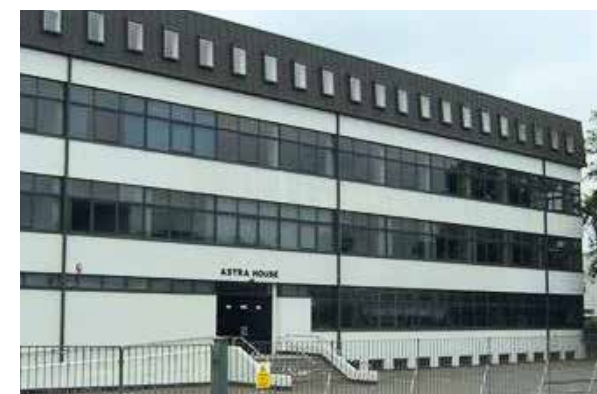
Astra House, Harlow
